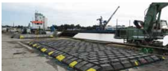
Sample of concrete mattress protection
